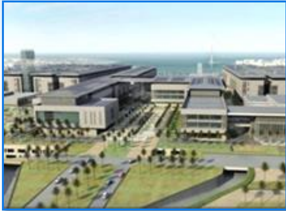
AL MUTLAQ BUILDING
